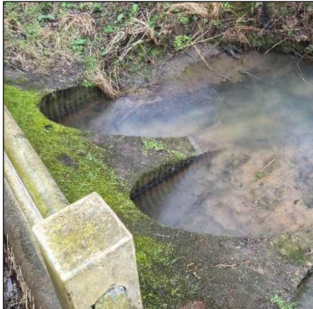
Figure 2-3 Broadwell Brook Culvert outlet under A361
