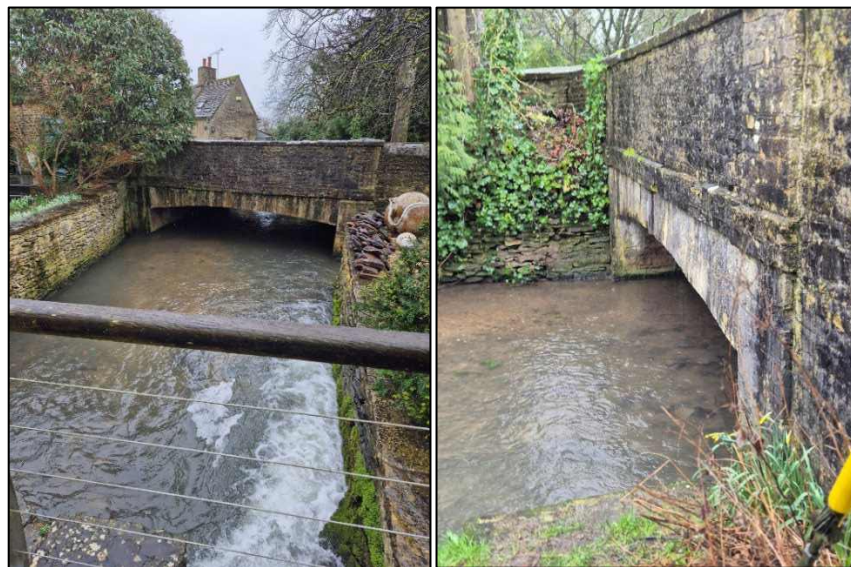
Figure 2-10 B4477 Bridge (Left: view upstream; Right: view downstream)
