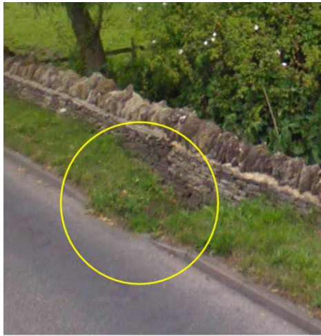
Figure 2-9 Highway drainage (Google images, 2016) (Left: Dropped kerb with no apparent outfall; Right: Hole through wall acting as outfall)
