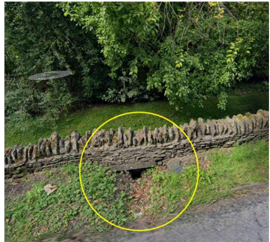
Figure 2-9 Highway drainage (Google images, 2016) (Left: Dropped kerb with no apparent outfall; Right: Hole through wall acting as outfall)
