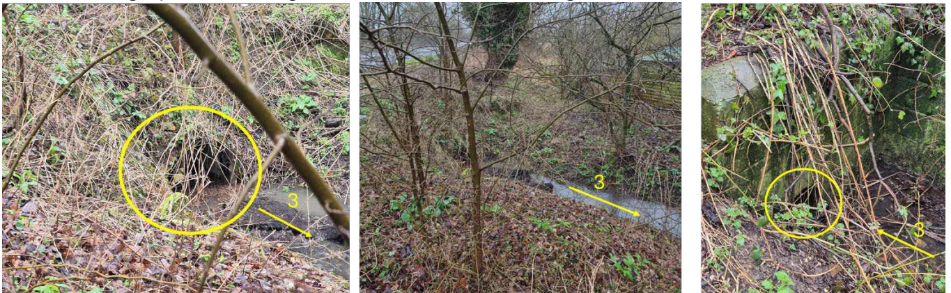
Figure 2-4 Watercourse 3 at the A361/B4477 Junction (Left: Culvert under A361 outlet; Centre: open channel; Right: Small diameter inlet.)
